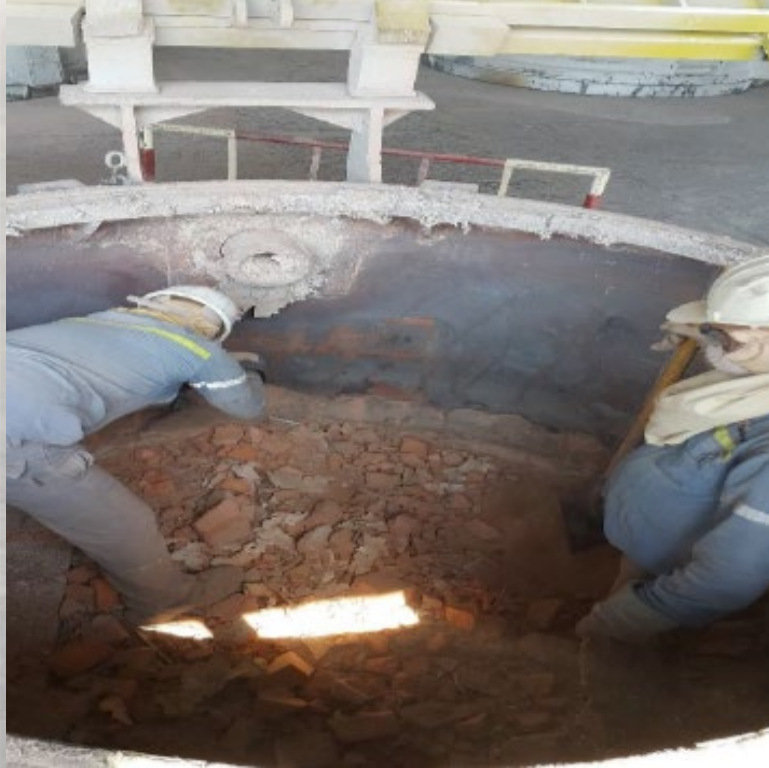
Metal Crucible Demolishing & Relining
