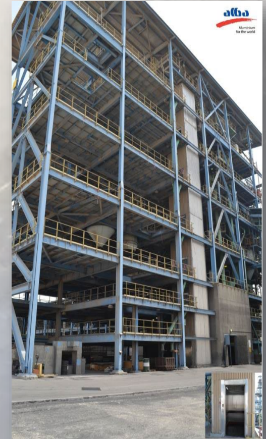
Heavy Goods Lift
