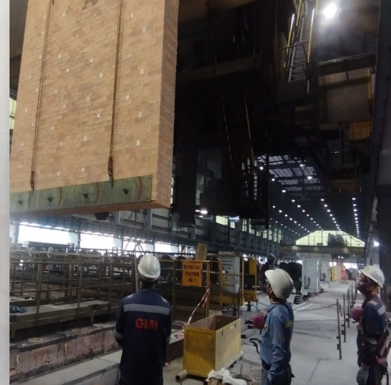
ABF Wall Building
